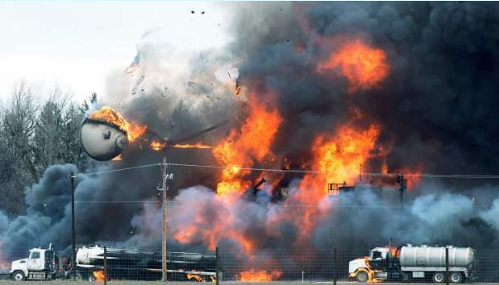
Result of a lightning strike of waste water facility near Greeley on April 17, 2015
